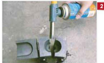
2 Preheat by butane torch to ensure the mould is totally dry every first joint regardless new or used mould
