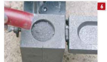
6 Pour a recommended size of weld metal into the mould crucible Check for leaks of weld metal Repeat step 4 in case of leak
