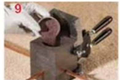
6 Pour a recommended size of weld metal into the mould crucible Check for leaks of weld metal Repeat step 4 in case of leak
