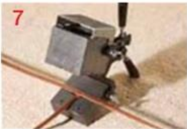
4 Fit conductors and ground rod snugly into the mould and lock the handle clamp Always make sure the mould is in a level position
